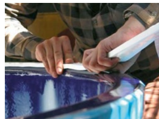
Installation of GORE® Gasket Tape Series 1000
